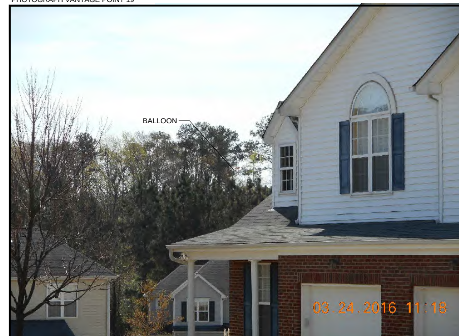
PHOTOGRAPH LOOKING SOUTHEAST. (APPROX. 2,505± AWAY FROM TOWER CENTER.) (BALLOON VISIBLE)
