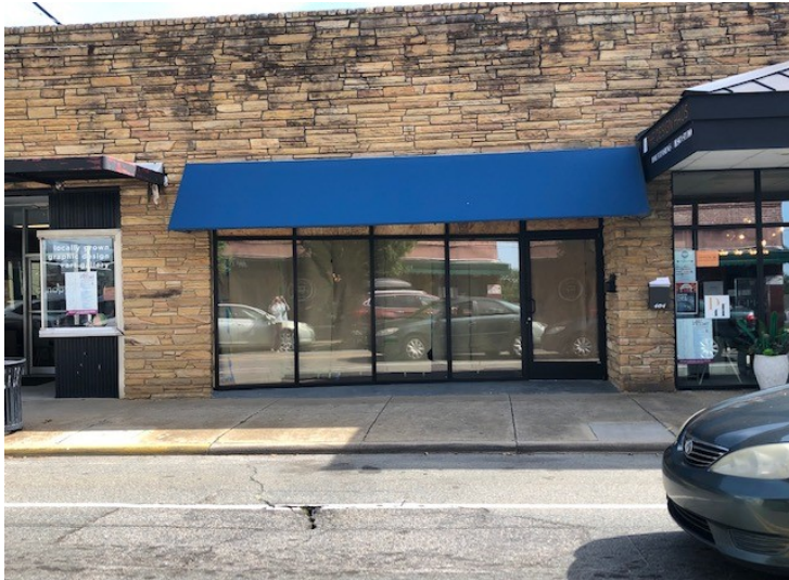
Work in Progress (August 2019)
