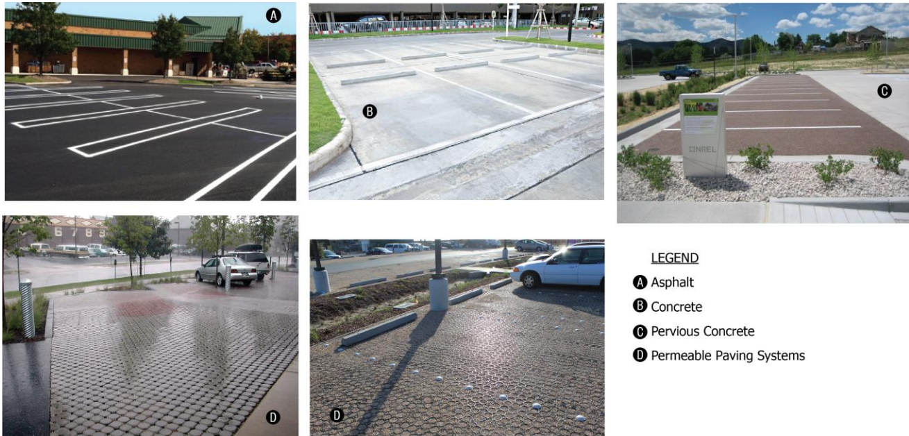
FIGURE 6.9.7.M: PARKING LOT SURFACE MATERIALS
