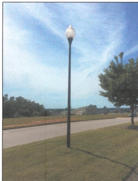
18' BLACK FIBERGLASS POLE WITH ACORN STYLE LIGHT COVER
