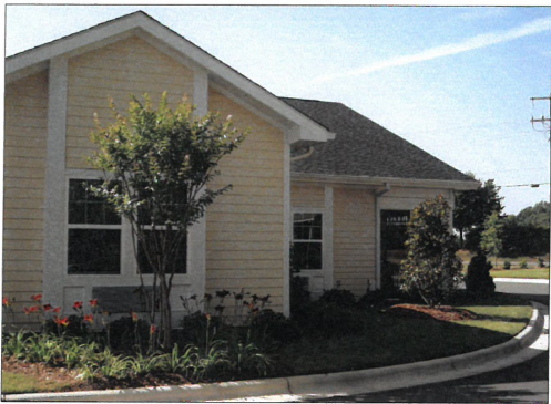
End of building wing
