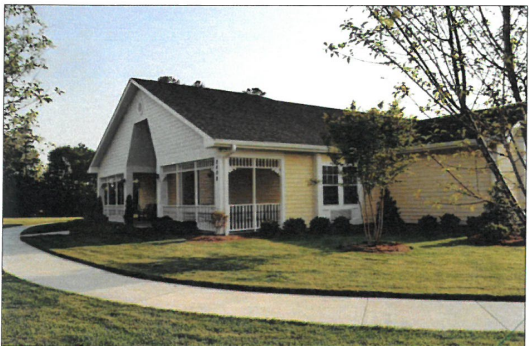
End of building wing
