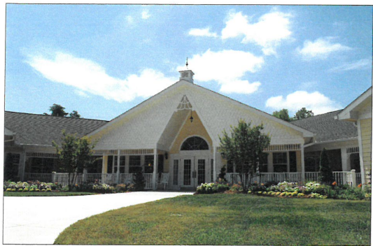
Carillon Assisted Living – Main Entrance
