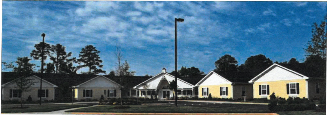
Front of building
