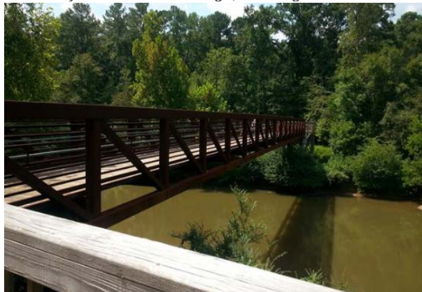
The Clayton River Walk Bridge, crossing the Neuse River
