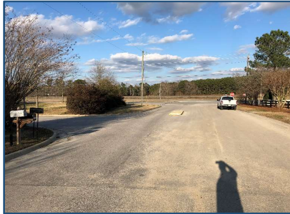
Northbound Approach of Hardee Lane at US 70 Business
