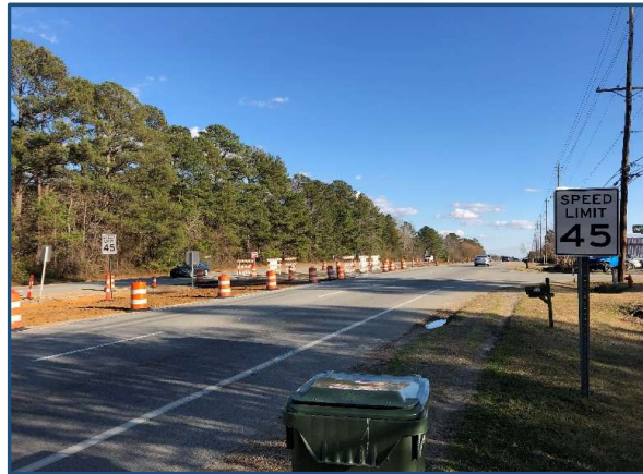
Eastbound Approach of US 70 Business at Astor Street
