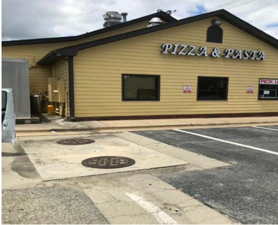
1000+ Gallon Gravity Grease Traps
