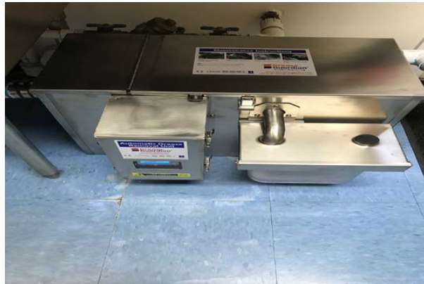
Automatic Under the Counter Grease Trap
