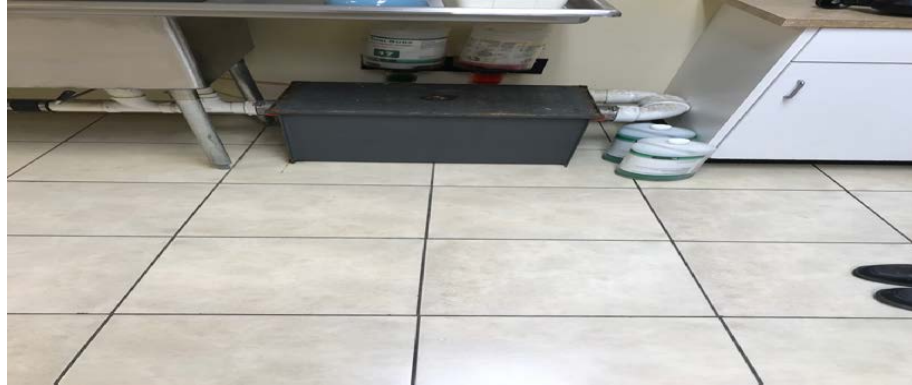
Automatic Under the Counter Grease Trap
