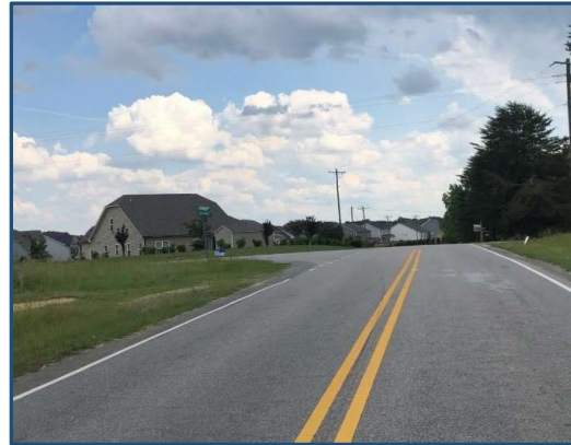
Southbound Approach of Glen Laurel Road at Vinson Road
