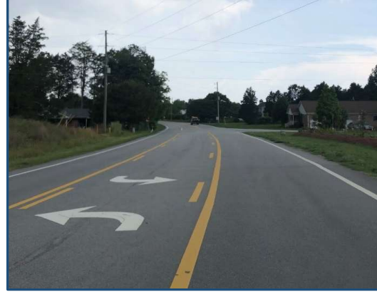
Westbound Approach of Powhatan Road at Glen Laurel Road
