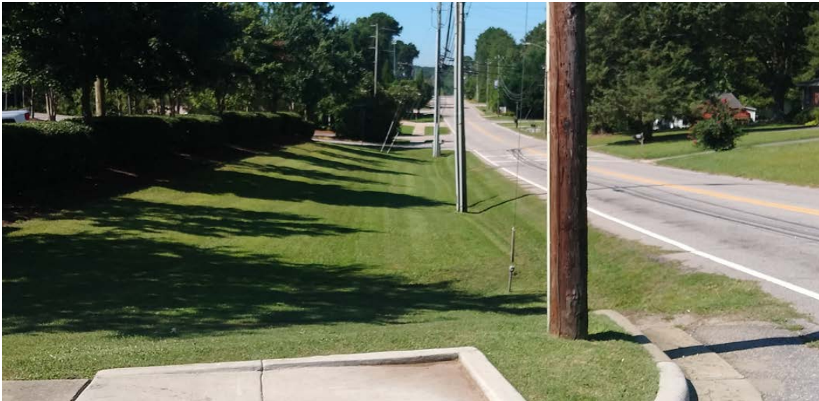
Ample space to complete the sidewalk gap south of Horne St
