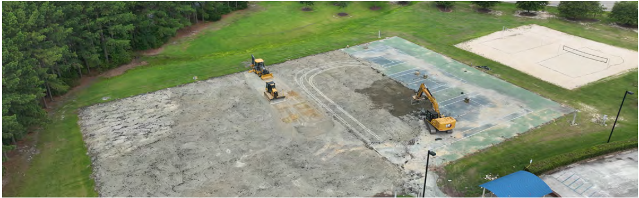
Park renovations are underway
