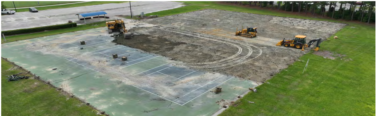
Demolition of older features has occurred
