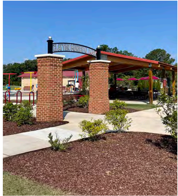
The entrance into Municipal Park could also serve as a trailhead for the community-wide greenway
