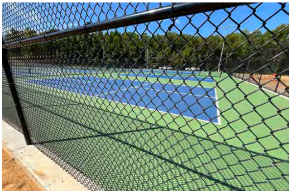
New pickleball courts at Clayton Community Center - photo by Town of Clayton
