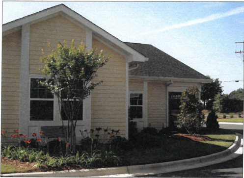
End of building wing
