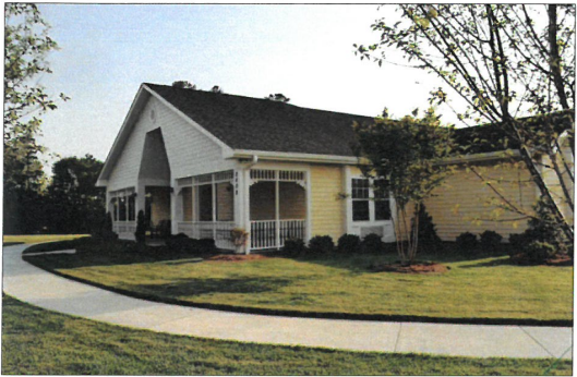
End of building wing
