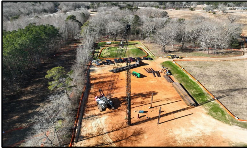
Image 8: 2026 Aerial Photo of the W. Clayton Elevated Water Storage Tank Construction
