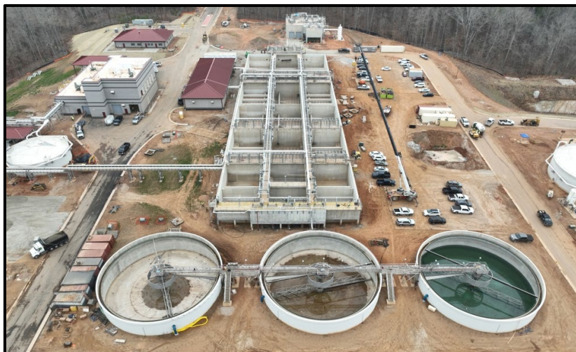
Image 7: 2026 Aerial Photo of Sam's Branch Water Reclamation Facility
